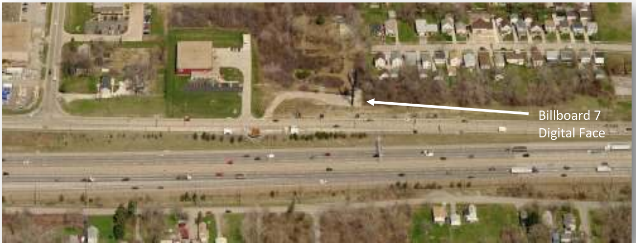
Figure 19. Oblique Aerial of Digital Billboard 7 on I-480
